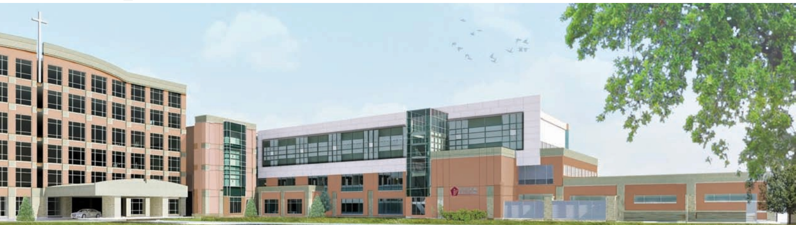
St. Mary Medical Center's expanded surgical department will feature 12 large surgical suites and four minor procedure rooms designed to allow for flexibility of equipment placement, ease of use and accessibility for surgeons and staff.
